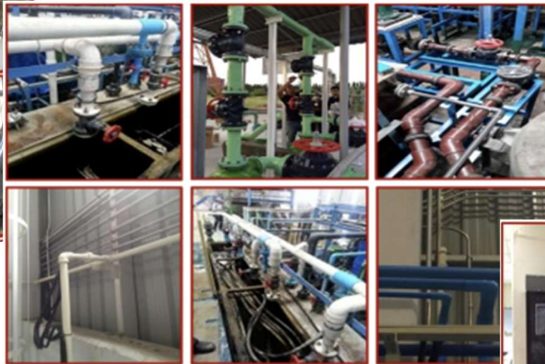
Installation Pipe System
