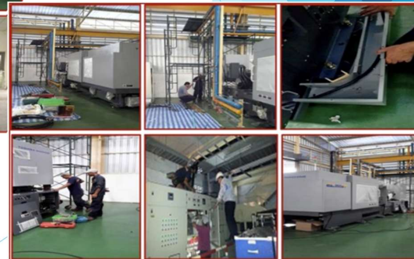
Installation electrical for full system
