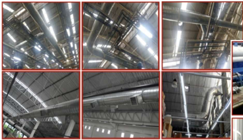
Installation Pipe System
