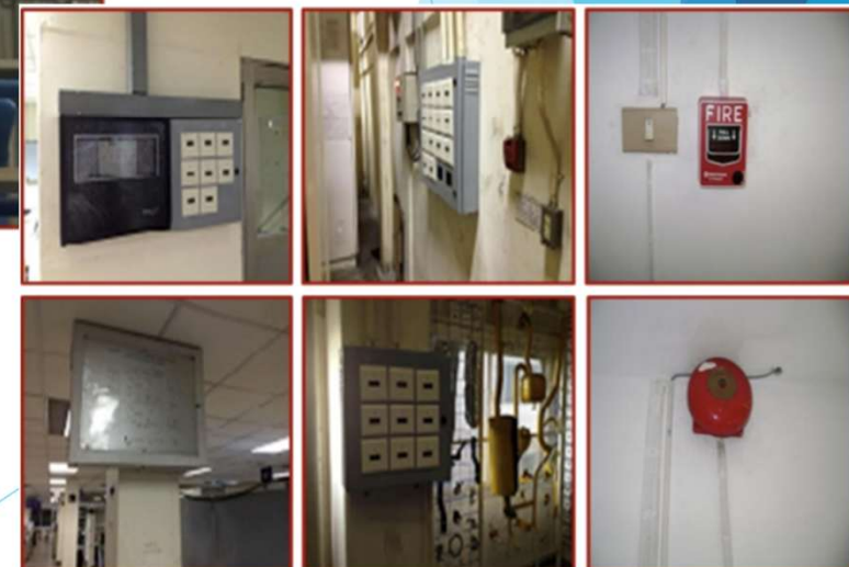
Installation Fire Alarm
